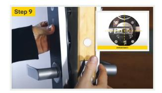
Taking care not to pinch the cables, fit the external furniture to the door. Ensure the spindle is aligned and sits in the latch when installing both the internal and external furniture to the door. For doors without a spindle (<45mm), ensure that the clutch spindle is fitted into the latch as shown.
