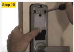
Using a Phillips screwdriver and selected mounting screws, fix the two handles together. It is now time to install the batteries in the lock. IMPORTANT: Do not close your door prior to installing the batteries or you could be locked out.
