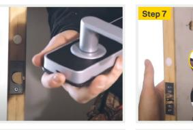
To fit the internal furniture to the door, feed the main cable and the DPS cable through the top hole and then fit the lock into place. Connect the DPS from the internal furniture to the DPS cable fit previously through the door.
