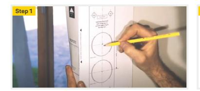
Using the door template provided, mark out the required holes for drilling including the latch and Door Position Sensor (DPS) hole. Then drill holes with appropriate tools.
