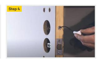
Insert the DPS through the 12.5mm hole on the door edge. Feed the cable first through the DPS hole.
