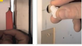
Align the DPS location onto the door jamb using a pencil. Drill a 12.5mm diameter x 15mm deep hole. Fit the DPS magnet into the door jamb. Mark the position of the latch bolt to determine the striker height. Fix the strike box to the jamb and then secure the strike plate over with the timber fixing screws. For lock setup, please refer to the Yale Access Quickstart Guide.
