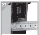
• Measure the door thickness and halve it.
