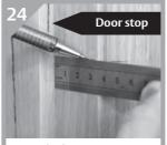
From the door stop along the horizontal line, measure and mark a vertical line at half the door thickness
