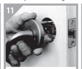
Position lever assembly (side with screws) so that it operates downward to retract the latch bolt.
